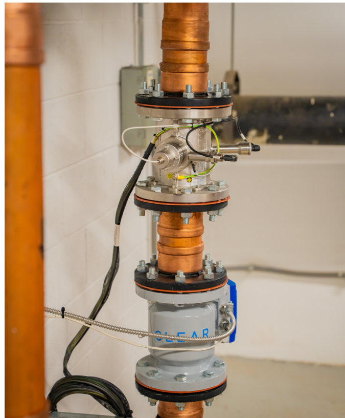
Figure 3. Close up of the HOD UV reactor (above) and flow meter (below).
