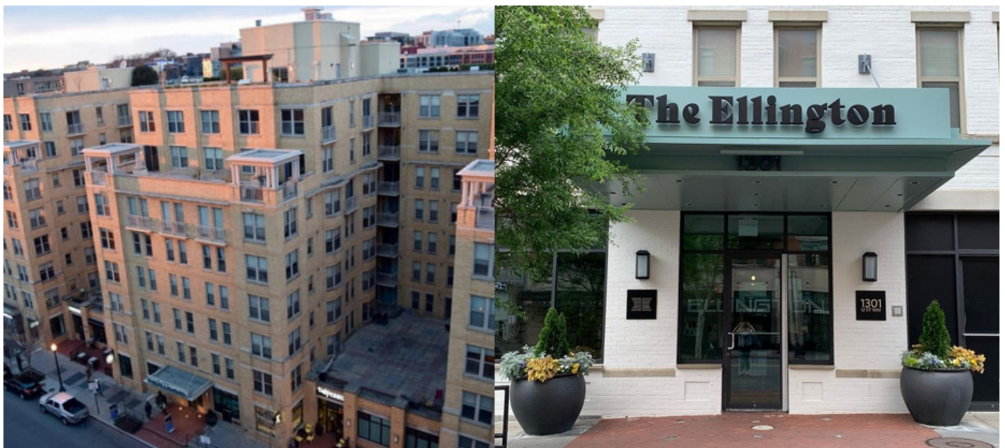
Figure 1: Exterior view of The Ellington
